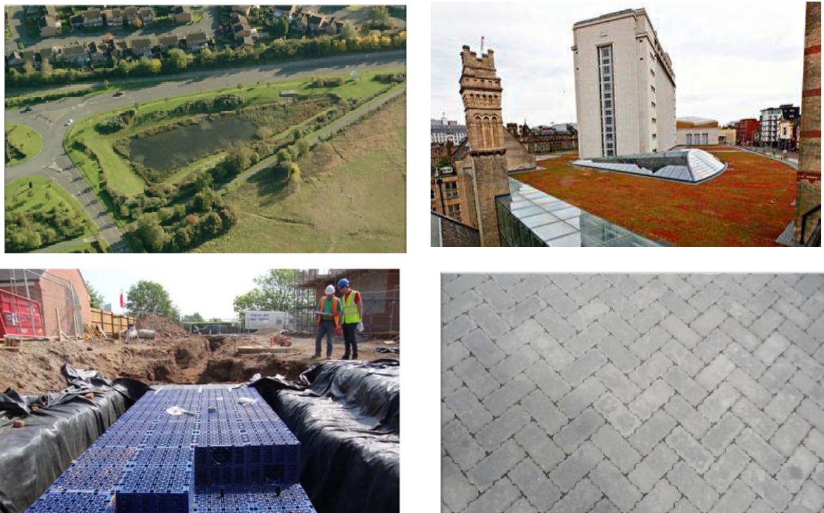
Figure 4-5: Examples of SuDS schemes that have been installed in Nottingham Top left: Attenuation basin at Nottingham Business Park; top right: green roof at Nottingham Trent University; bottom left: geocellular units at Ruddington Lane, bottom right: example of permeable paving
